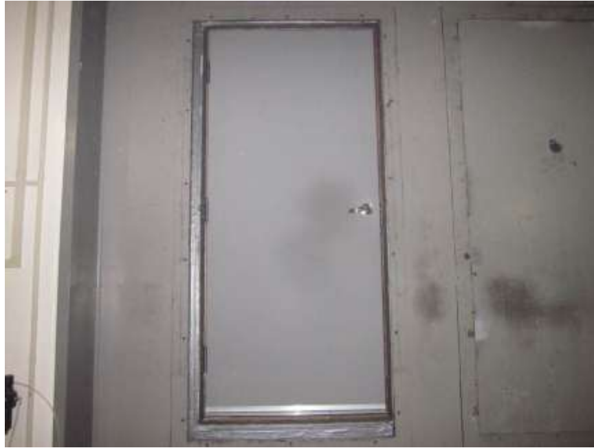
Receive Room View of Installed Test Option B
