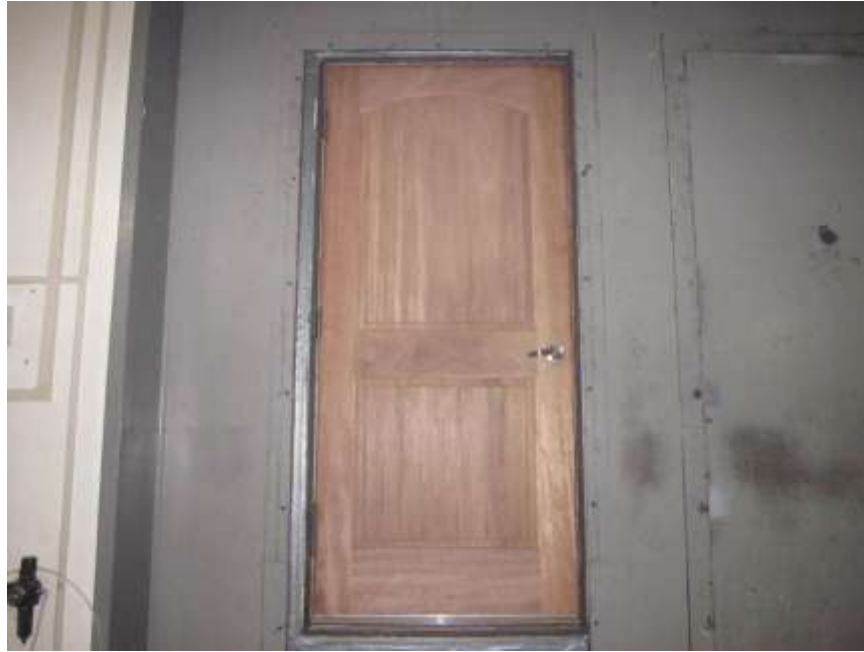
Receive Room View of Installed Test Option A
