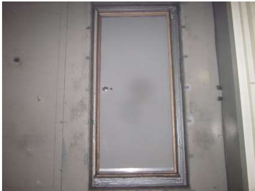
Source Room View of Installed Test Option B
